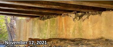
Paint Fork Bridge foundation (rusted steel and crumbling foundation)
